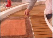
Dry-fit the hatch again, using extra care. Make sure that the lines in the decking on the hatch line up perfectly with the lines on the surrounding PlasDECK:
