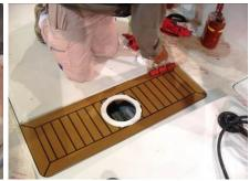
Clean any excess glue with a clean rag and denatured alcohol as soon as possible:
