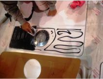
Finish spreading the glue. Then carefully lay the panel into the glue and use the floor roller on it:
